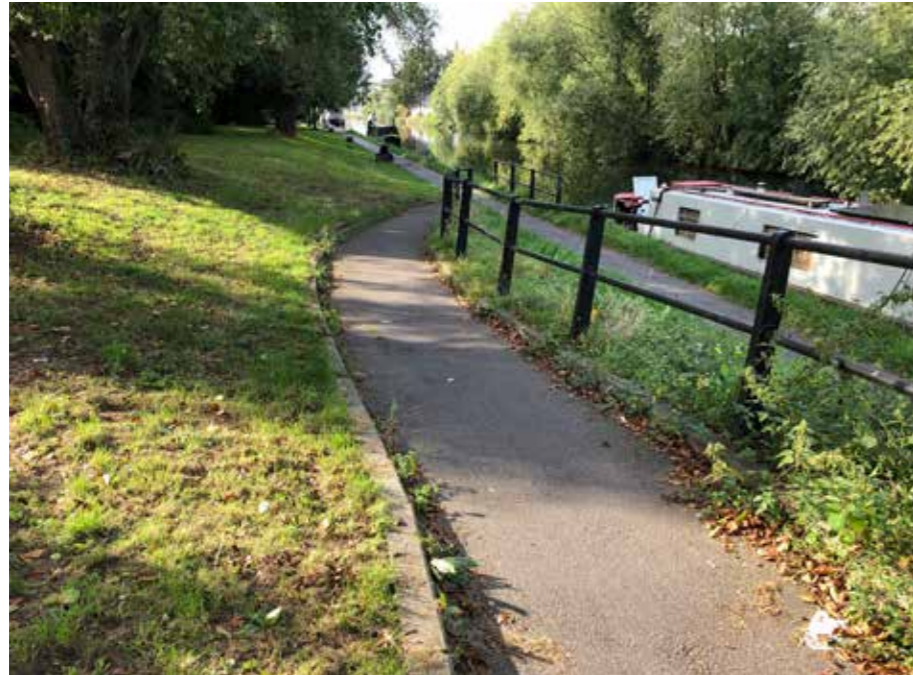
A hardstanding with seating built into landscape opens up towards the canal and the towpath ramp.
